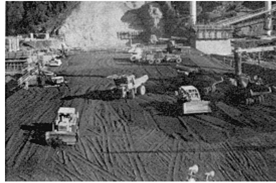
Figure 1-6. RCC placement operation
