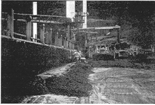
Figure 1-11. Placement of conventional concrete facing
