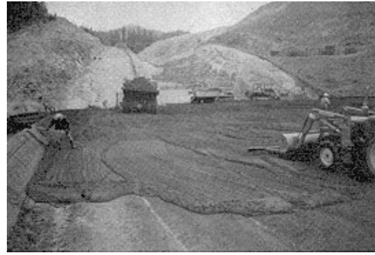
Figure 1-8. Application of mortar bedding
